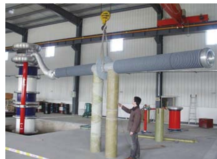
Testing Wall Bushing
