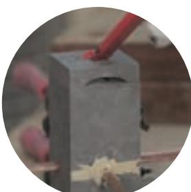
6. Close the lid of mould & from the side ignite the starting powder with the flint gun.
