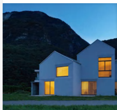
Backup Power with ESS 2kVA-72kVA
