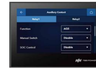
Generator AGS Control Setting
